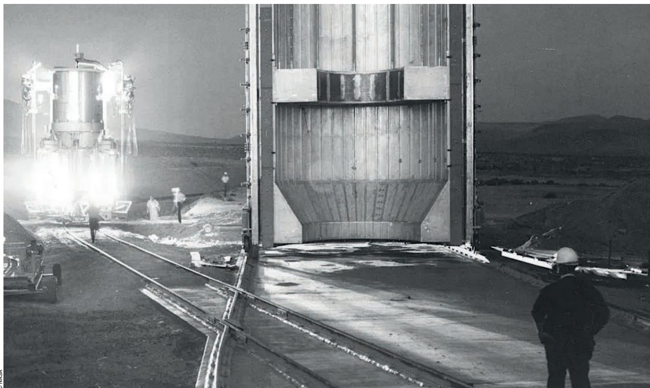
A nuclear-powered rocket engine from 1967, more accurately called a Nuclear Thermal Rocket, preparing for testing. While often associated with E=mc^2 , this design primarily utilises the heat from nuclear fission to create thrust, not direct mass-energy conversion
