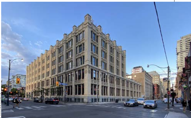
This Neo-Gothic building, clad in terra-cotta, stands at 299 Queen Street West in Toronto. It houses the headquarters of Bell Media, the media division of Bell Canada
