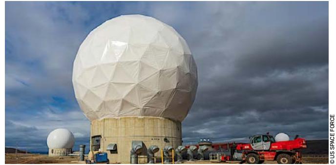
Radar dome at Pituffik Space Base
