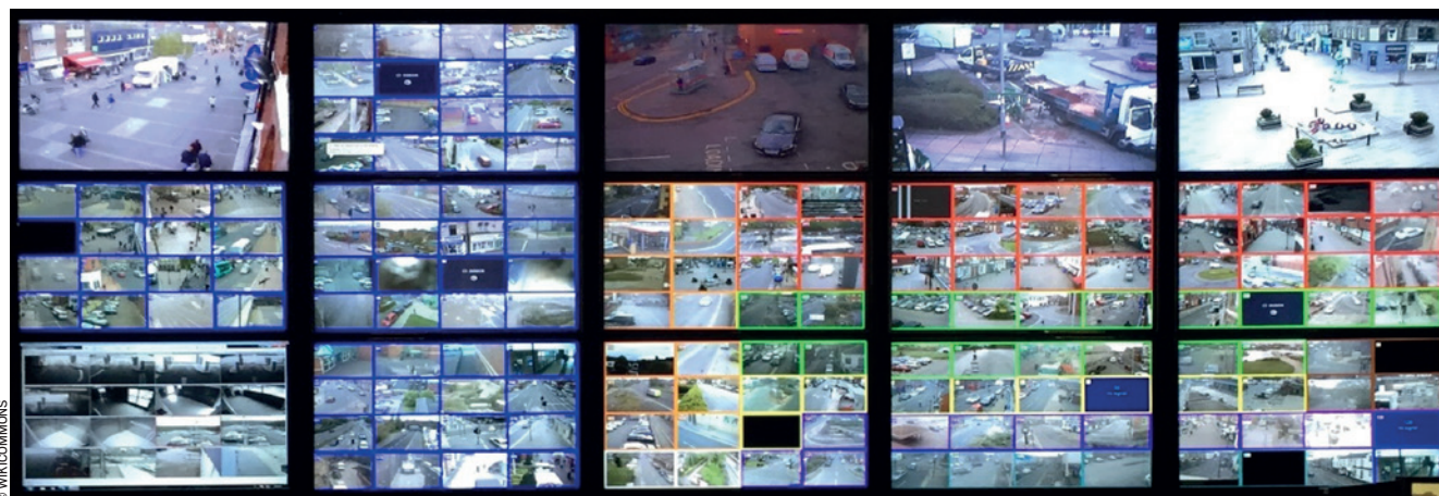
A monitor wall with fifteen 42-inch monitors for 176 on-street cameras in a public space CCTV control room
