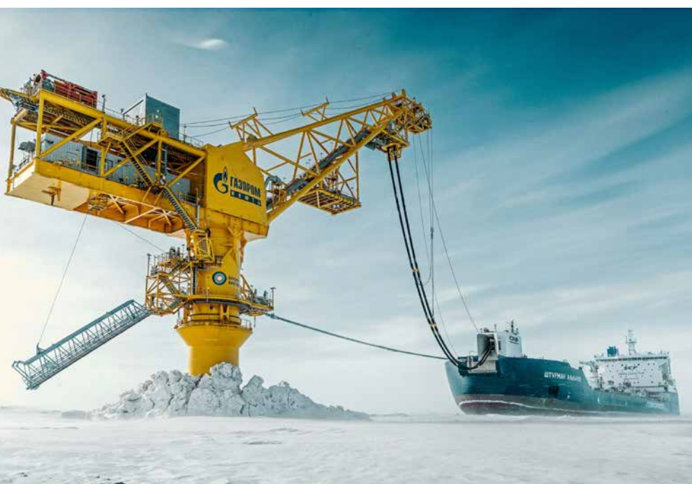
Articulated Loading Column at the oil and gas terminal in Novoportovskoye, Russia
