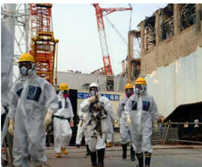
IAEA experts depart Unit 4 of TEPCO's Fukushima Daiichi Nuclear Power Station on 17 April 2013 as part of a mission to review Japan's plans to decommission the facility
