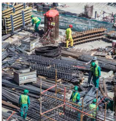
Workers at a construction site in Dubai. Foreign direct investment is an important source of capital for infrastructure projects
