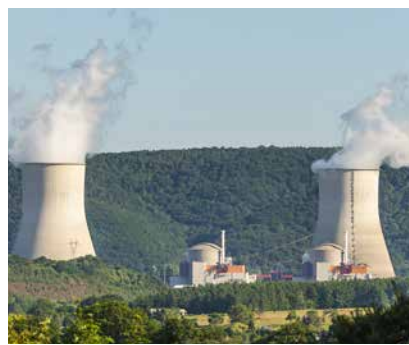
Nuclear Power Plant, Chooz France
