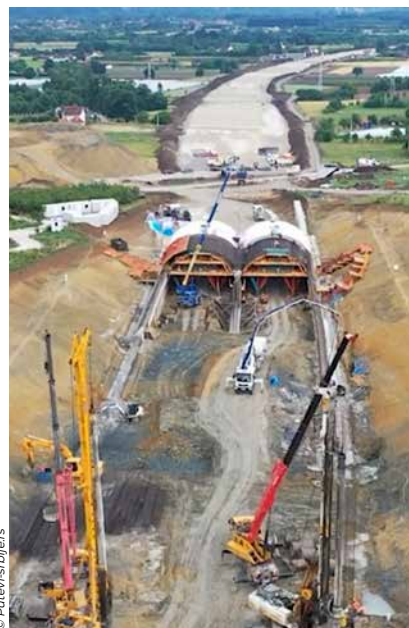
© Putevi/Srbijers Construction of motorway E-763 section, Preljina-Požega
