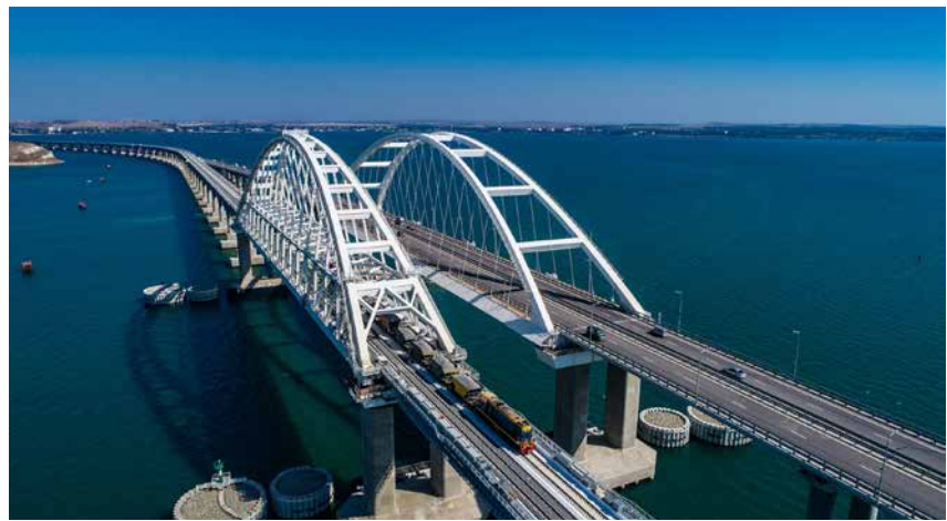
The Kerch Bridge, linking Crimea to Russia
