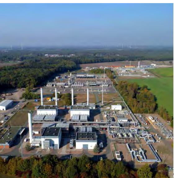
Gazprom's UGS natural gas storage facility in Rehden, Germany
