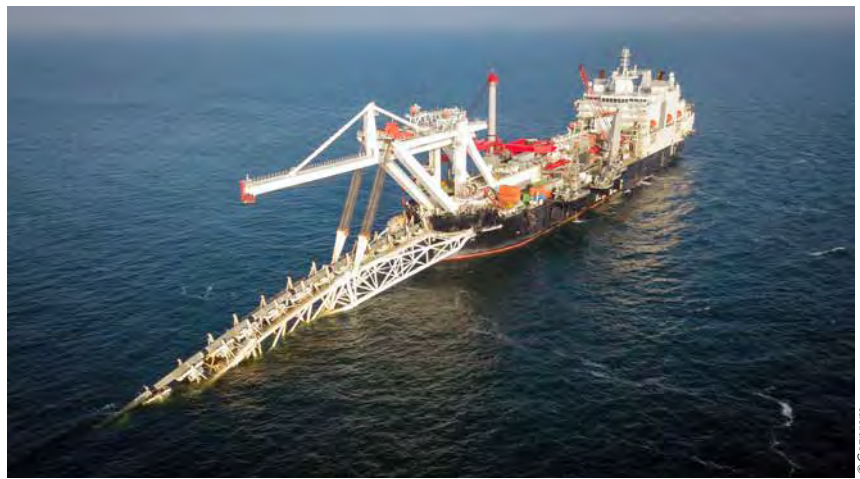
Pipe laying operations in German territorial waters
