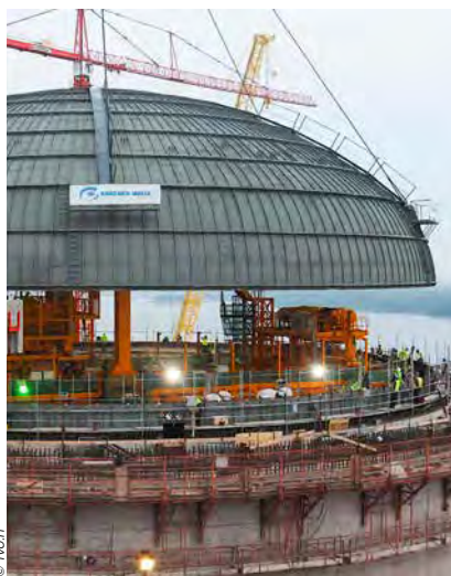
Lifting of the steel liner part in November 2009
