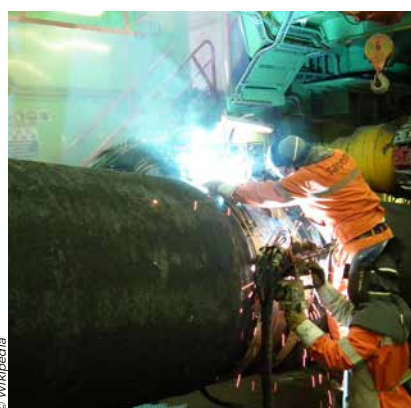
Two pipes are welded together on the Castoro Sei pipelaying vessel
