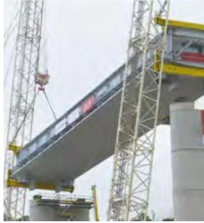
assembly of the parts. The deck will be completed by the slab, made with prefabricated elements in reinforced concrete and subsequent finishing casting.
