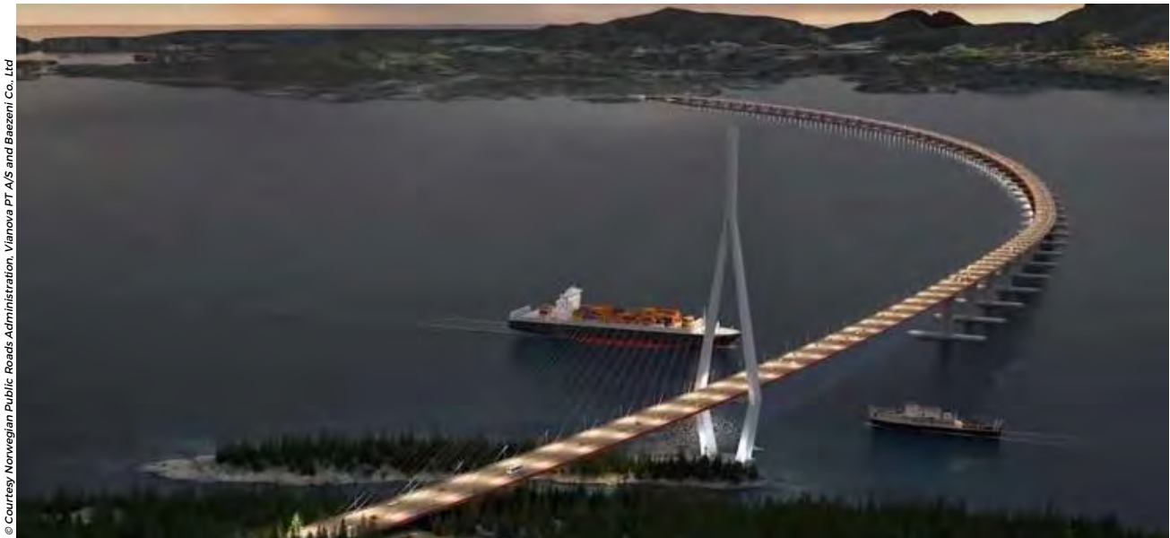
A floating suspension bridge that has been proposed to cross Norway's Bjornafjord
